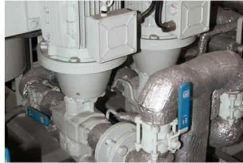
1 Redundant gear pump units KF
