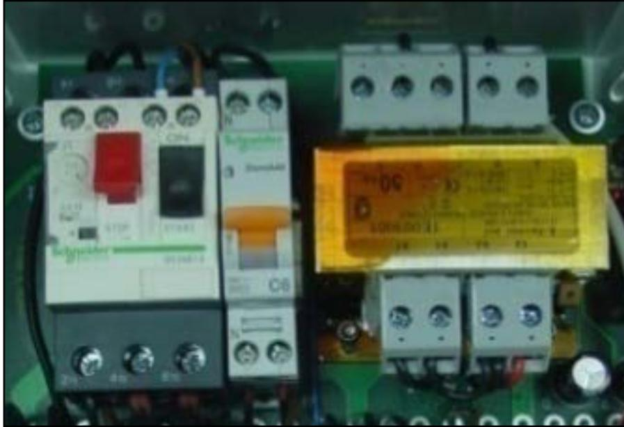
**Fig. 9.4.5 – Mother Board – Switch breaker (inside Main Control Box)**
