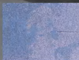
ISO Wa 2/SSPC-NACE WJ 3 Thorough Cleaning
