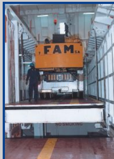
Cargo lift 50 t SWL.
