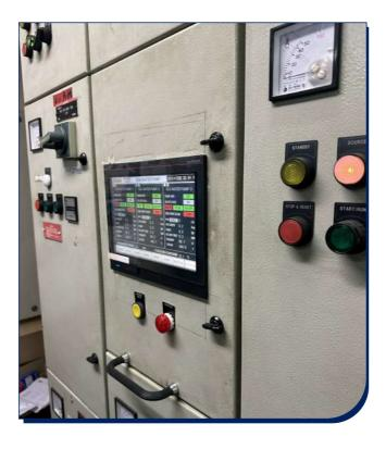
**3. Redundancy Concept:** The dual-PLC configuration embodies a 100% redundancy concept. In case of any issues with the primary PLC, the
