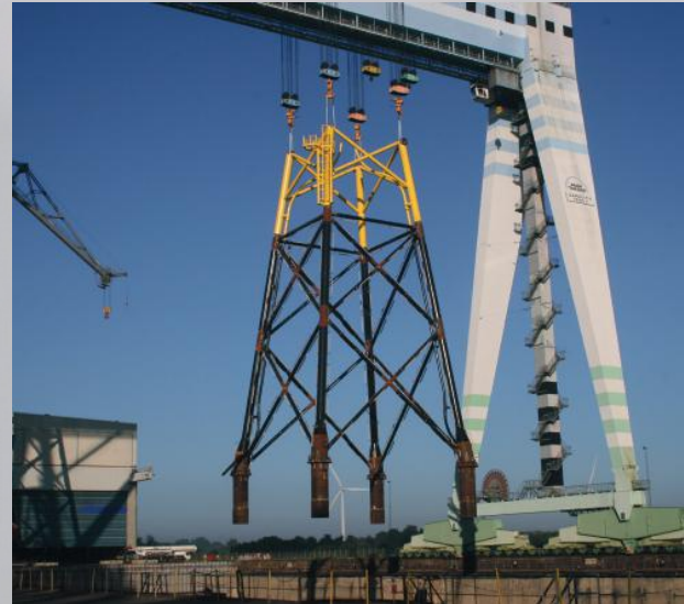
Wind turbine foundation
