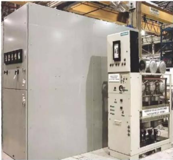
Footprint comparison (MV AIS & MV GIS - only equipment size considered)
