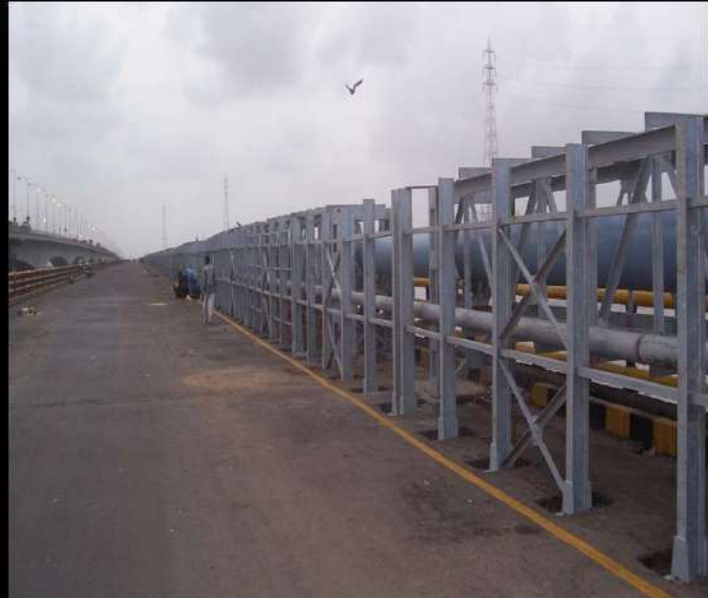
1.5 KM Long Pipe rack at Vashi bridge for GAIL [Project:- Dhaej-Uran gas pipeline] Manufactured, transported and erected at site including core drilling on concrete
