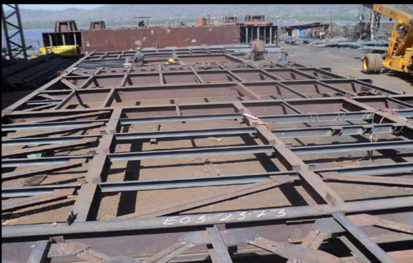
1.5 KM Long Pipe rack at Vashi bridge for GAIL [Project:- Dhaej-Uran gas pipeline] Manufactured, transported and erected at site including core drilling on concrete
