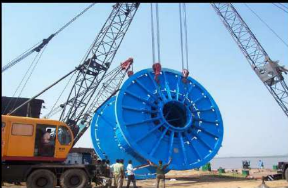
Lifting of Cable reels onto barge
